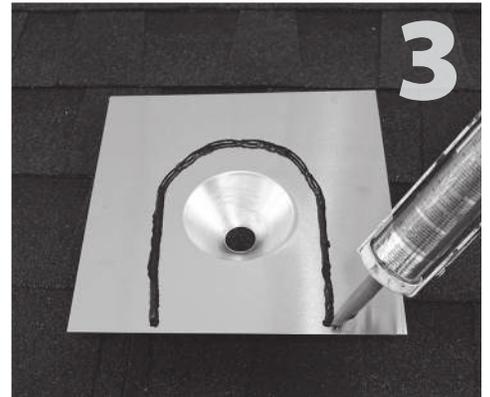
Apply sealant compatible with the roofing material on the underside of the flashing in an upside down U.
