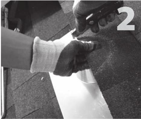
Slide flashing (item 1) into position centering the flashing hole with drilled hole. Remove any nails that prevent getting the flashing into position. Using a hook blade, cut shingle around cone to allow correct placement of flashing. Flashing should not hang over bottom (drip) edge of shingle below.
