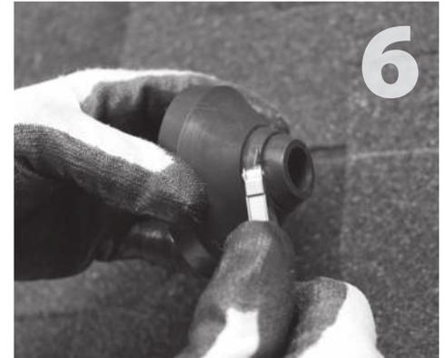
Cut EPDM collar (item 2) to appropriate conduit size (see Drawing 1, Detail A on reverse). Take care to cut a clean, level line.
